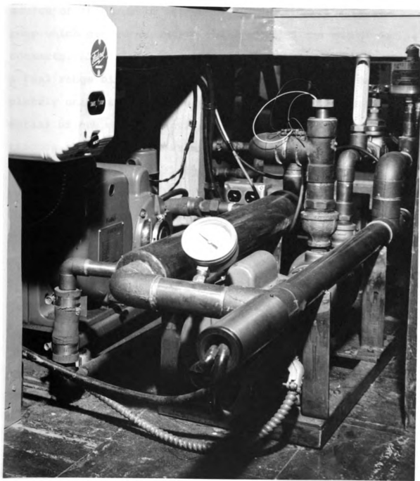
Figure 20. Focusing Coil Temperature Control System. The Pump and the Heat Exchangers.
