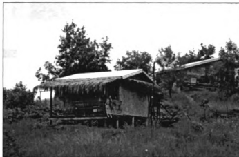
Figure 5 - House: One Story, Sawali Walls & Corrugated Iron Roof
