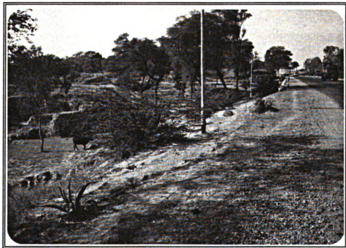
Deficient Access Control - Specific Paths: Hazardousness Evaluated by MOH [SPATHS].
