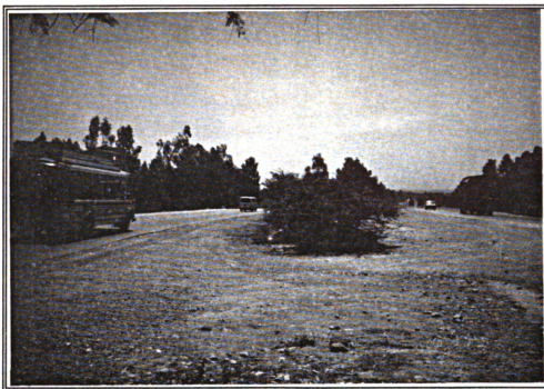
Deficient Access Control - Median Openings: Hazardousness Evaluated by MOH [MEDOPN].
