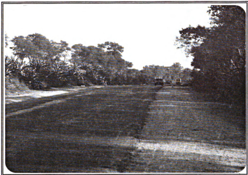
Deficient Pavement Markings: Hazardousness Evaluated by MOH [PMARKS].
