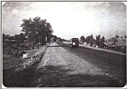
Deficient Pavement Width: Hazardousness Evaluated by MOH [PWIDTH].
