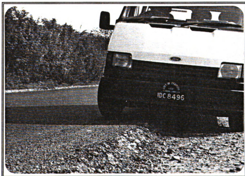
Pavement Condition Rating: Hazardousness Evaluated by MOH [PVCOND].
