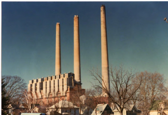
Figure 18. 6 x 8 inch reduction of the original 8 x 10 inch color print of the Eckert Station Plant.
