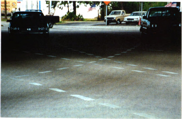
Figure 5.5: Pavement marking overlap creates driver confusion.
