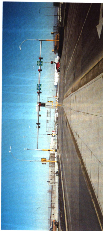
Figure 5.1: SPUJ with cross-road going over the freeway with all signal heads located on a single overhead tubular beam.
