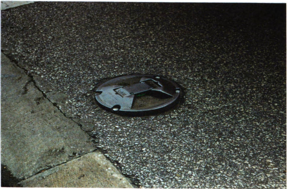
Figure 5.6: "Runway" lighting to help illuminate the turning path. Note the buildup of debris.
