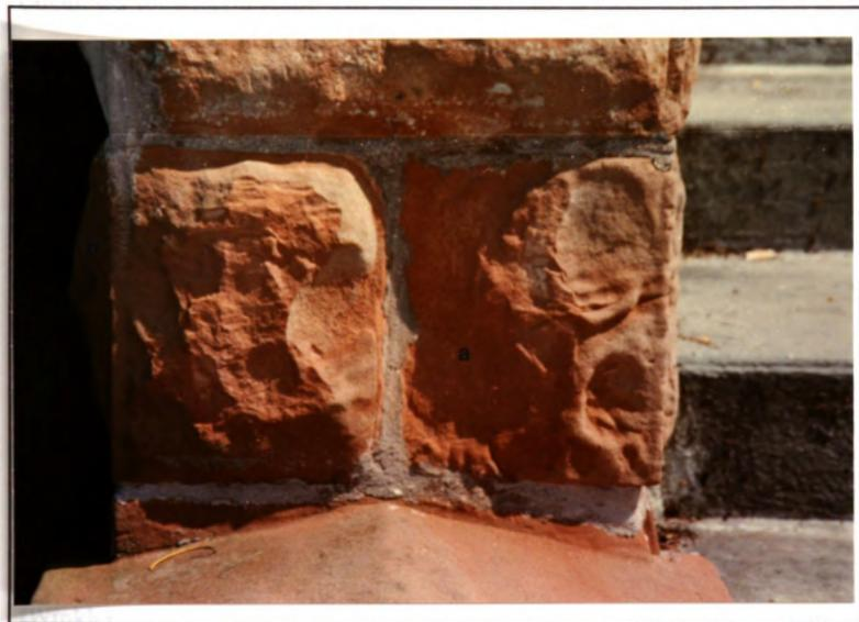
a) Large indentation weathered into a sandstone block at Morrill Hall. Note the depth of the indentation. b) Example of the non-uniform, convex fashioning of the sandstone blocks.
