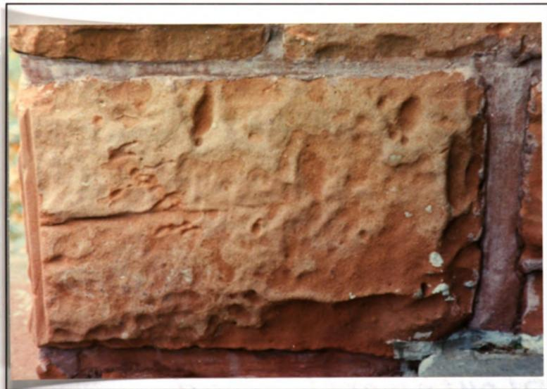
Small indentations (incipient honeycomb weathering) created by salt efflorescence at Morrill Hall.
