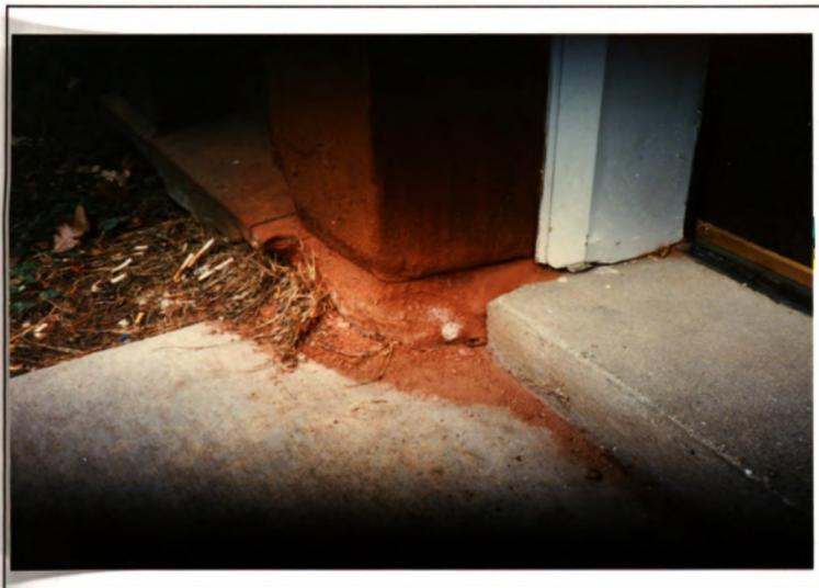
Eroded pillar showing the maximum height of capillary rise in the sandstone at Morrill Hall. The black line on the pillar marks the maximum height (approximately 8 inches).
