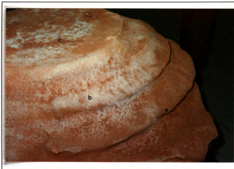
Weathered pillar base from Morrill Hall. The picture shows a) the destruction of the decorative sculpturing, b) the efflorescence build up and c) the grit/loess development.
