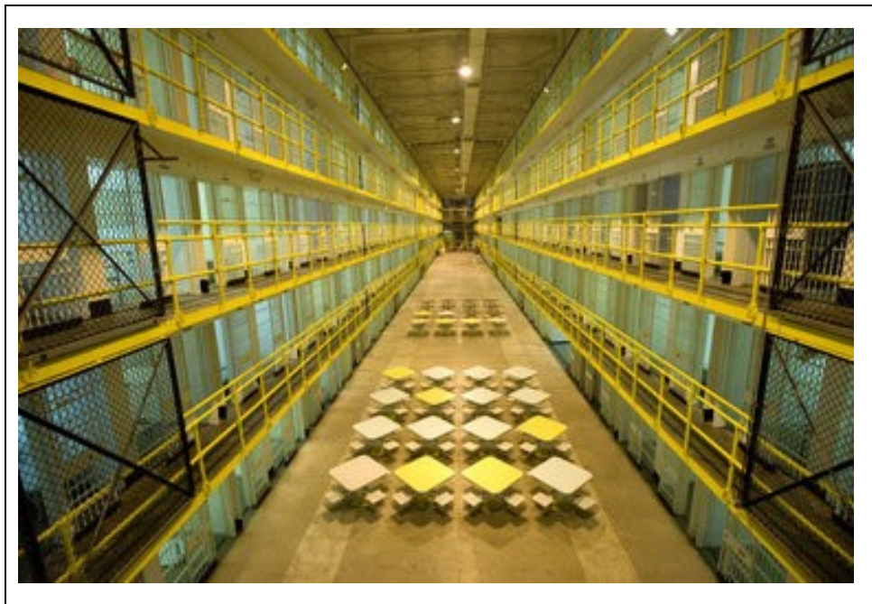
Figure E-2. Parnall Correctional Facility Cell Block 7 (Photo credit: Nick Dentamaro - Jackson Citizen Patriot)
