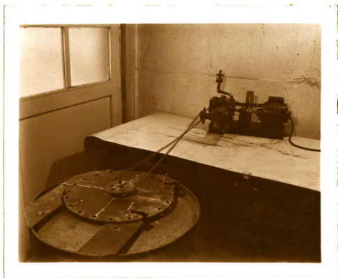
Fig. 4. Sprinkler-rotating mechanism.
