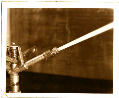
Fig. 22. Jet of water issuing at 40 psi from a \frac{1}{4} inch diameter circular orifice with a 6 diameter extension tube.
