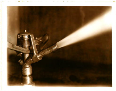
Fig. 38. Sprinkler with 7/16 inch diameter tube 1\frac{1}{2} inches long operating at 40 psi.
