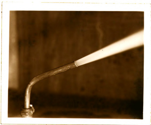
Fig. 40. Jet of water issuing at 40 psi from a \frac{5}{16} inch diameter tube with a 3\text{-}\frac{1}{4} inch diagonal portion.
