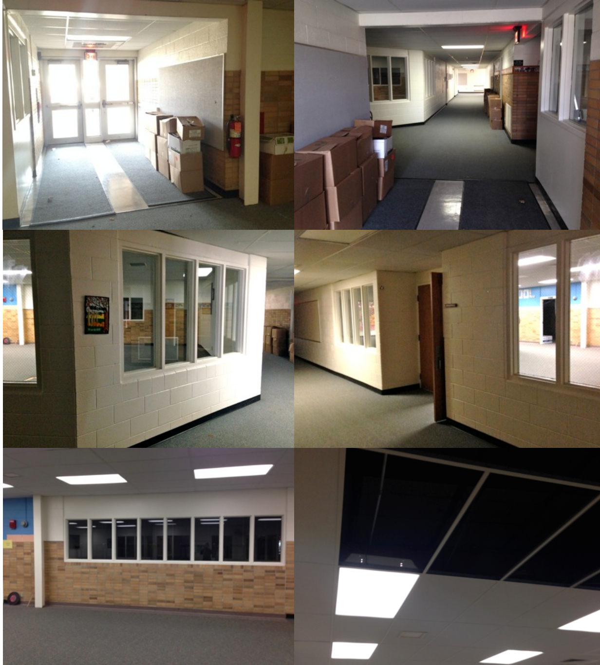
Figure 6: West entry with window to office (top left), front entry (top right), view of media space (middle left), concrete block and blue low-pile carpeting (middle right), brick and concrete block in media space (bottom left), missing acoustical ceiling panels (bottom right)
