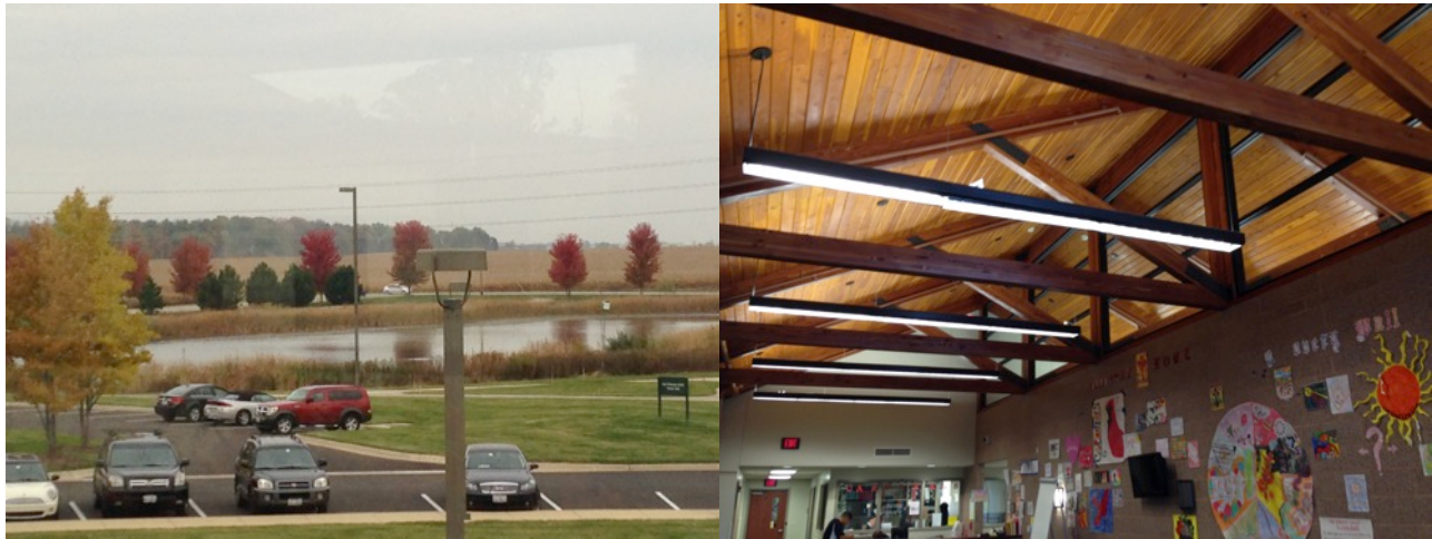
Figure 26: View from second floor corridor (left), wall does not meet ceiling in resident lounge (right)
