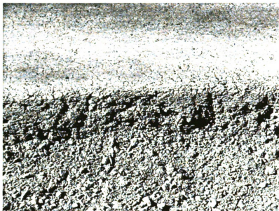
Figure 10. Edge View of RCC Pavement (After One Day).
