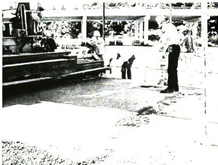
Figure 5. RCC Being Placed and Tested for Density Before Rolling.
