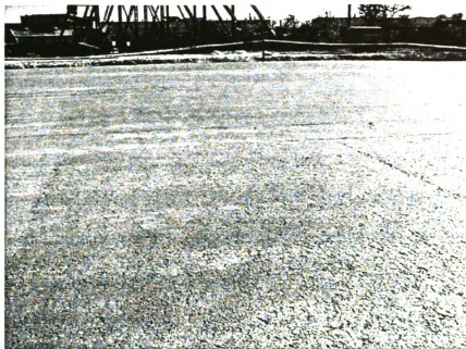
Figure 8. Far View of RCC Surface (After One Day).
