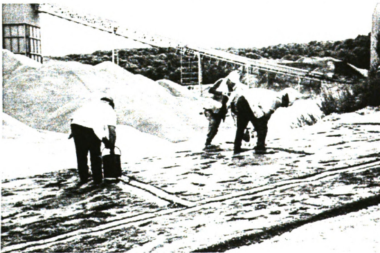
Figure 37. Inducing of Joints Using the Vibrating Fin in an RCC Base.
