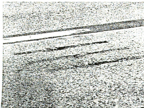
Figure 51. View of Spalling in Grout Covering of M-14 DBR Site.
