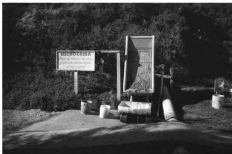
Figure 6. Fine Screen (Hydrasieve)*.
