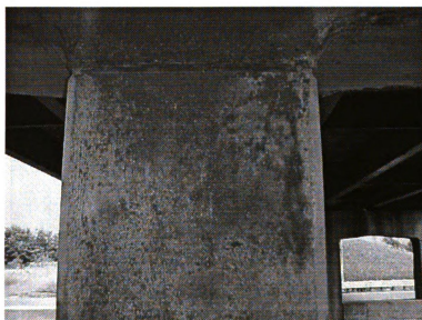
Figs. 5.2 Column condition after surface repairs
