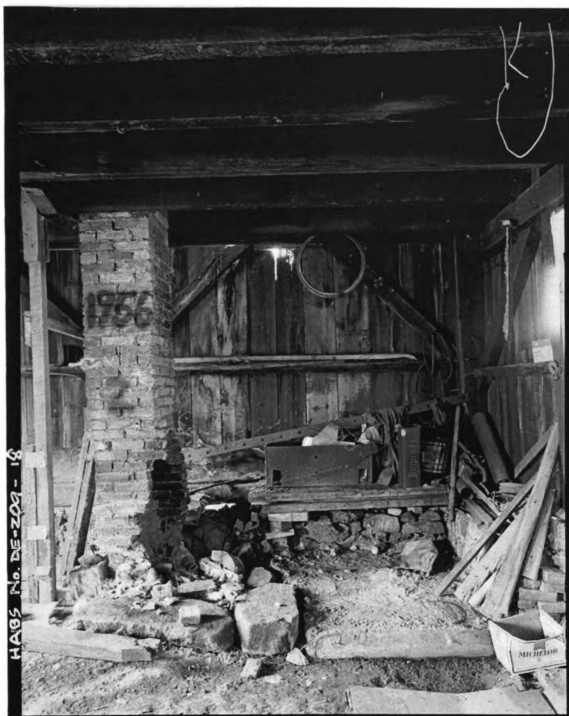
Figure 33. Wilson Alexander Agricultural Works Complex. First Floor Forge Hearth Remains. (DE-209-18).
