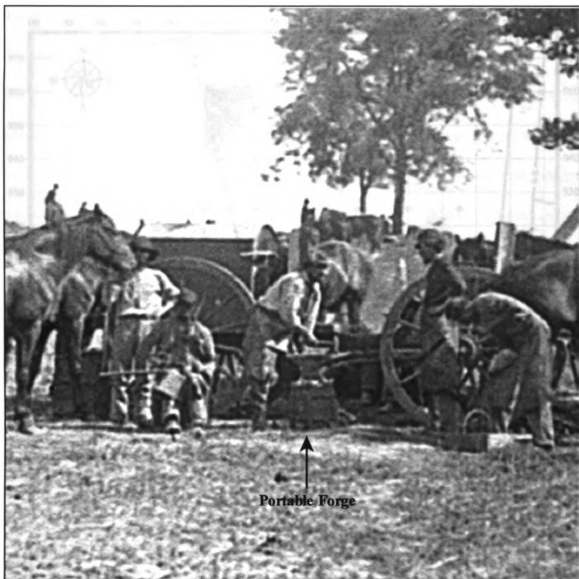
Figure 26. An Example of a Portable Union Blacksmith Shop.
