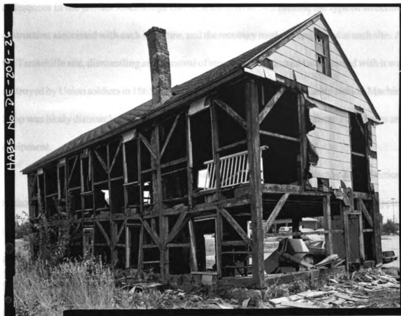
Figure 39. Wilson Alexander Agricultural Works Complex. Structural Frame Revealed During Demolition. (DE-209-26).
