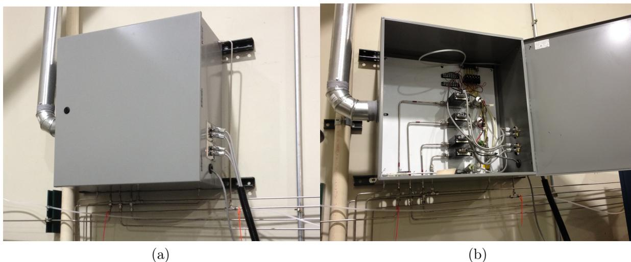
Figure 2.3 (a) Photo of the DS6 gas line connection ventilation box, with the front door closed (b) Photo of the DS6 gas line connection ventilation box, with the front door open, showing the mass flow controllers and isolation valves inside.
