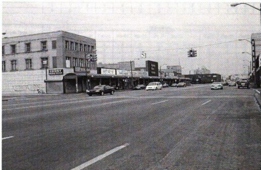
Figure B.2 – Woodward At Milwaukee After Improvements
