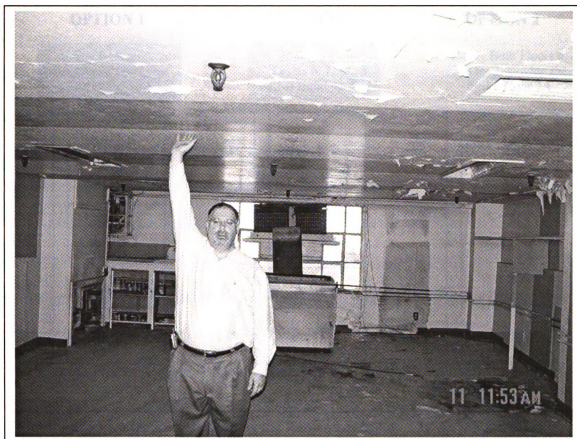
Figure 21: Seventh Floor Level of Building A with Low Ceiling Height of Just around 7 Feet, Making it Not Compliant with the MBC Minimum of 7'6"
