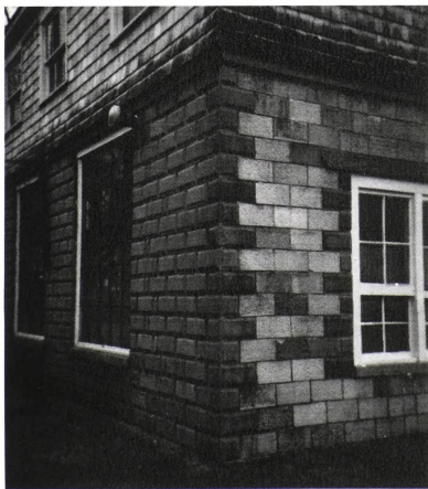
Figure 4.29: Garage, brick construction detail (Photo taken by author).
