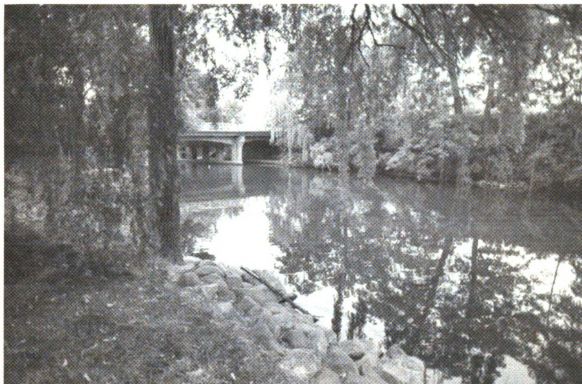
Figure 3-1. View of the Farm Lane Bridge over the Red Cedar River from the USGS Gauging Station on the Campus of Michigan State University.
