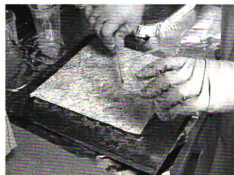
(f) Wet out of bottom mat layer
