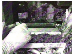
(j) Placement of top material layer
