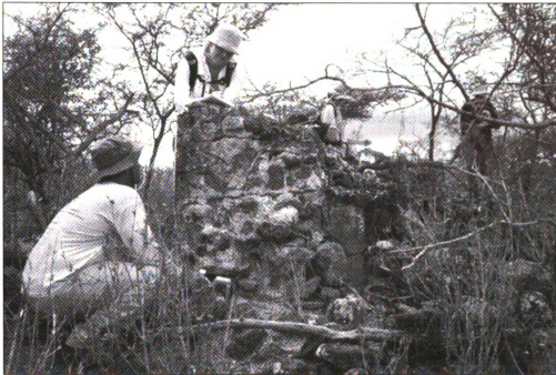
Figure 5-17. Documenting boiling train at Long Pt. Road site, SJ9KR5/22-1. The structure had been built up in three crude masonry courses, finished in dressed stone and plastered. Pictured: Bart Beecroft, Texas A&M, and Krysta Ryzewski, Brown University.
