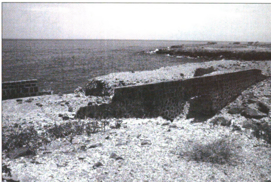
Figure 5-6. Coast round island road in lower St. John parish. Between White Hall and Dogwood estates SJQ19. Torrents have gushed through the ghut this bridge spans and have undermined its foundation. Continuing easterly around the island the road vanishes altogether.
