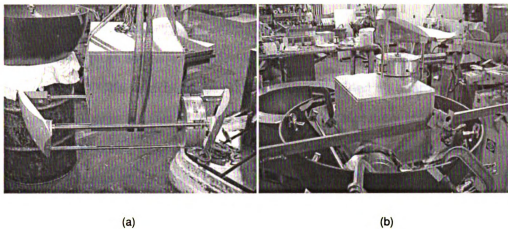
Figure 6.2. Steps taken during the propulsion mechanism installation, (a) shows the alignment box with the first axis, (b) shows the first axis installed, and the beginning of the axis two and three installation
