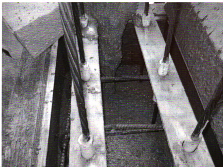
Figure 5-2 Casting of Pull-out Test Block
