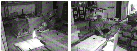
Figure 4-8 Release of Prestress – Both ends of the beam being cut simultaneously
