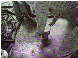
b) Step1 - Cone Filled with SCC
