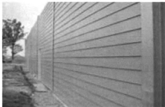
Figure 2.17 Sound barrier of wood-cement particleboard in Czech Republic (CETRIS, 2005)
