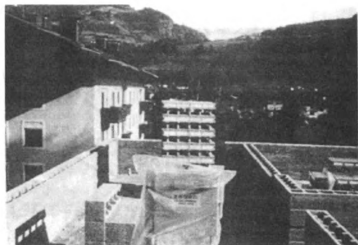
Figure 2.16b Exterior and interior walls with WCP blocks (Hoene, 1997)
