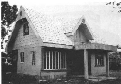
Figure 2.19 Wood strand cement board for all walls and sidings in Japan (Eltomation Company)
