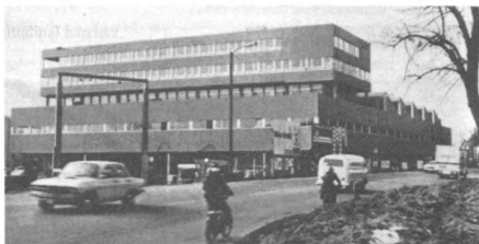
Figure 2.21 Wood fiber cement board as exterior-wall cladding of the Sandoz Laboratory in Basel, Switzerland, (Deppe, 1974).
