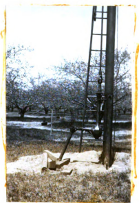
Figure 11. Power-take-off drive and speed reduction unit of Wind Machine Number Two
