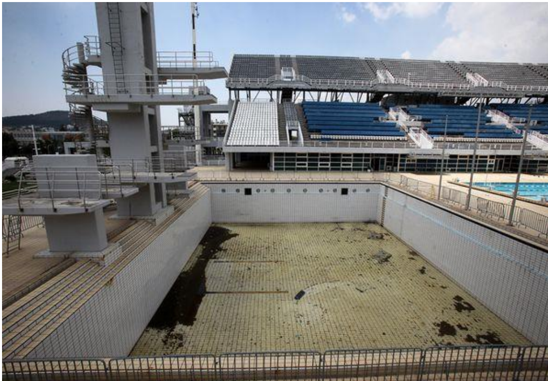
Figure 3 abandoned Athens Olympic stadiums
