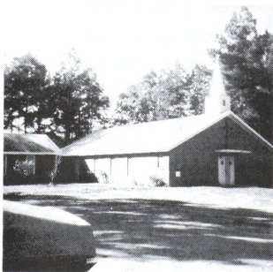
The new Mt. Zion CME Church, built in 1963. This is an evidence of change in the small town church on the East Texas landscape. Photo by author.
