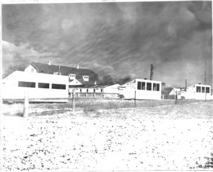
Figure 4. The three experimental houses used in the second trial. From left to right the houses are one-half double pane, single pane and double pane.
