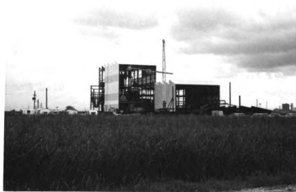
Figure 25. The partially completed shell of the Tinguaro sugar mill. Obsolete cane processing equipment, some of which can be seen installed in the building, led to the closing of the mill after the 1964 grinding season which was its only time of operation. Sugar cane grows in the foreground.
