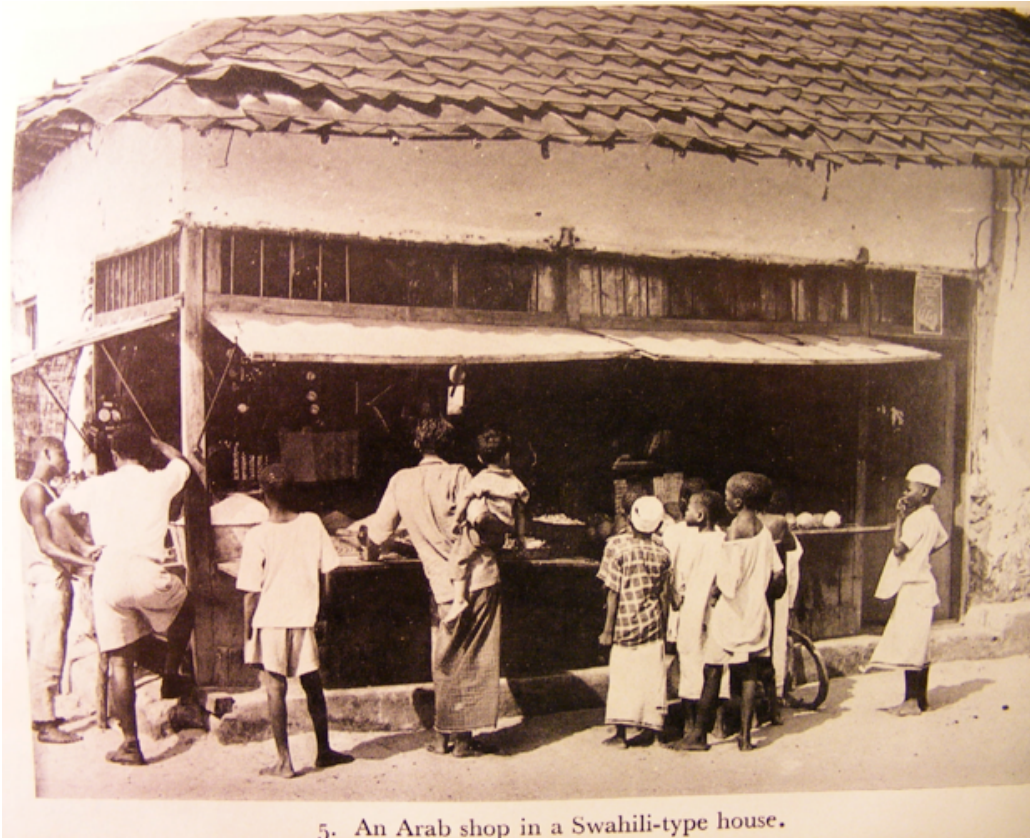
Figure 1.2: An Arab shop in a Swahili-type house in late-colonial Dar es Salaam. 170
