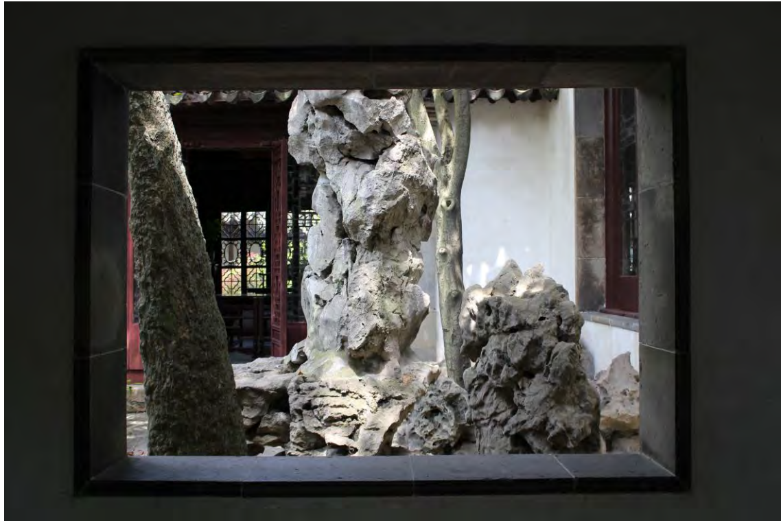
Figure 6: The wall openings framed by blackened terracotta create a “picture” of the plants or rockery. Lingering Garden, Suzhou. (Copyright ©2015 Yiwen Xu all right reserved used by permission).
