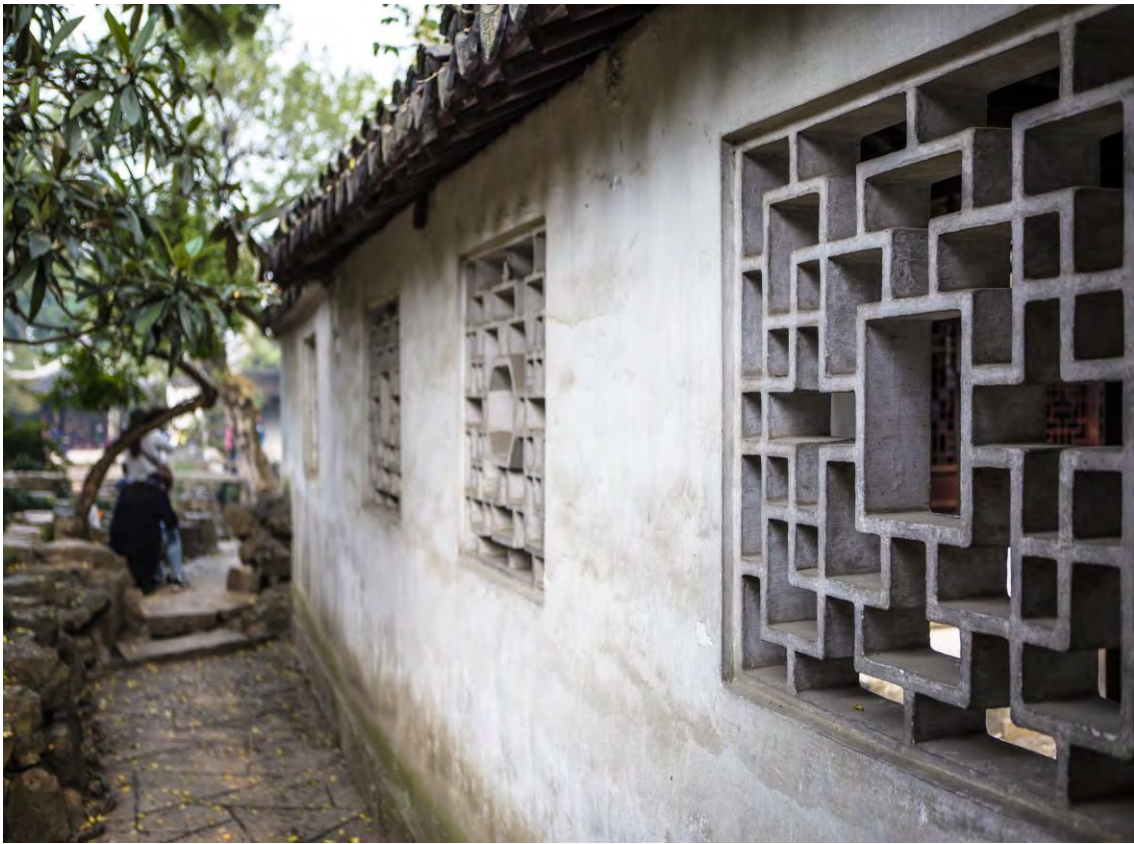
Figure 14: The whitewashed wall with lattice windows. Humble Administrator's Garden, Suzhou. (Copyright ©2014 Kun Zhang all right reserved used by permission).
