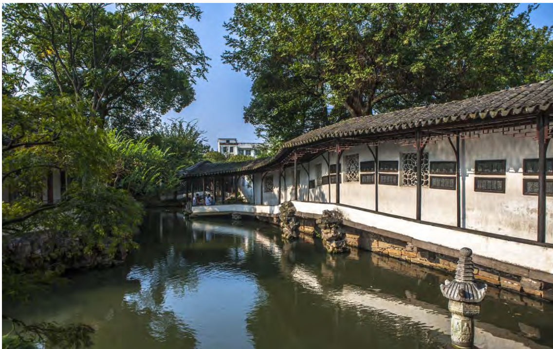
Figure 16: The double walkway built with a whitewashed center wall with lattice windows in the Humble Administrator’s Garden. (Copyright ©2014 Kun Zhang all right reserved used by permission).
