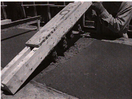
Figure 35. Removing Void Restraint From Finished Beam
