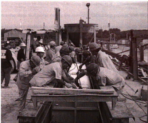
Figure 20. Installing Top Reinforcement On NCC
