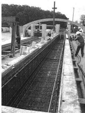
Figure 17. NCC Casting Bed Prior to Casting
