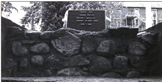
Figure D.2. The eastern foundation wall (Unit 11, N320 E320) demonstrating the fieldstone construction.
