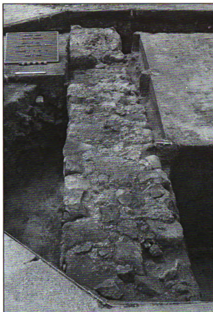
Figure 4.10. The northern foundation wall looking west. The wall measured 2.5 feet in width and was composed of large granite field stones joined with a coarse mortar (Units 9, 13, 23, 15; N 335 E315-330).
