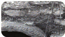
Figure 7.4: Failure of the Headwall due to Heavy Spalling
