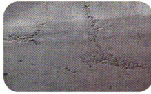
Figure 2.21: Honeycombing on a concrete surface (Source: http://www.arche.ps.u.edu/thinshells/module%20III/concrete_behavior_text_files/image020.jpg )
