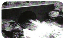
Figure 2.2: Culverts functioning as Inlet Control (Source: http://www.hydrocad.net/culvert1.htm )
