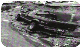
Figure 1.7: Failure of a 30 year old, 96" CMP in West Bountiful, Utah
