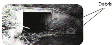
Figure 2.12: Debris at the opening of the culvert (Source: http://www.ctre.iastate.edu/pubs/tech_news/2005/mar-apr/debris-at-culvert.jpg )
