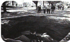
Figure 1.3: 84" Diameter CMP Failure in Maryland
