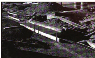
Concrete Paving of Earth Slopes
