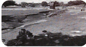
Figure 1.4: Failure of 126" diameter CMP in Charlotte, North Carolina
