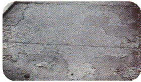
Figure 2.17: Scaling exposed on Concrete Surface (Source: http://www.pci-potomac.com/faq/scaling.jpg )
