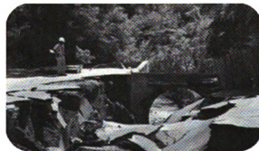
Figure 1.5: Failure of a 30 year old, 96" diameter CMP in Hickory, North Carolina
