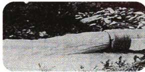
Figure 2.4: Culvert Flowing under Pressure Flow (Source: FHWA, 2001)
