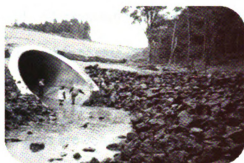
Figure 2.10: Riprap Basin to Protect Streambed and Stream Slope (Source: www.tankmasta.com.au/images/Rural/Culvert.jpg )
