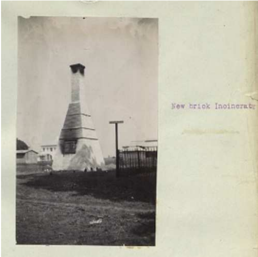
Figure 35: Refuse Incinerator, Bathurst
