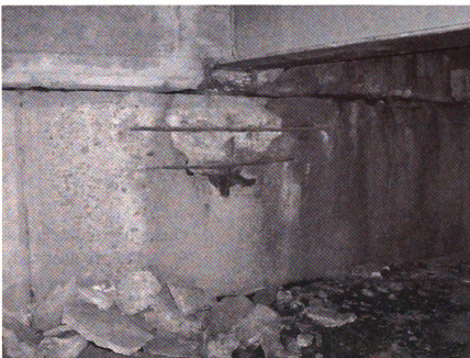
Figure 1-3 Concrete spalling in the abutment wall
