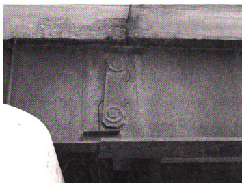
Figure 1-8 Corroded pin-hanger assembly
