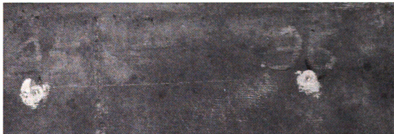
Figure 4-3 Brass cylinders installed on the abutment wall
