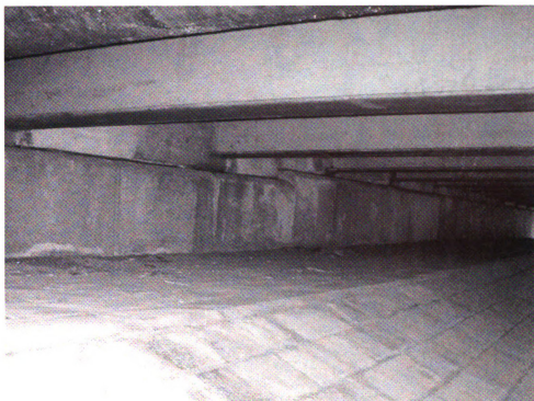
Figure 4-17 West abutment of bridge B2.1
