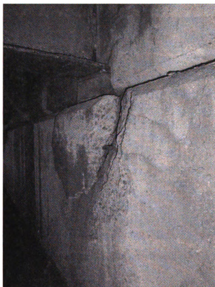
Figure 1-4 Pull-out of concrete block in the abutment wall under girder support
