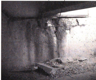
Figure 1-12 Concrete pullout caused by pavement pressure
