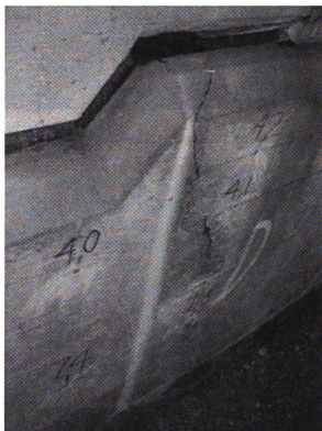
Figure 4-21 Abutment distress in bridge A1.7
