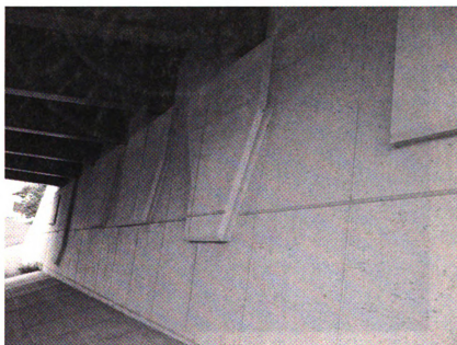
Figure 1-7 Repair of damage in abutment walls
