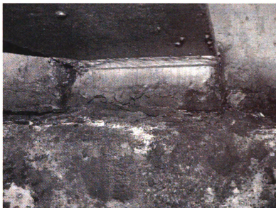
Figure 1-9 Water leaked to the abutment wall underneath a girder
