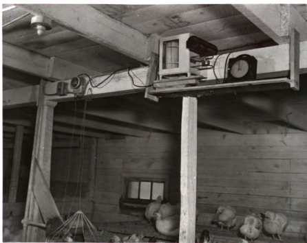
Fig. 65. The hygrothermograph and the time of operation instrument were placed approximately six feet from the floor or one foot from the ceiling in order to be out of the farmer's way and to avoid roosting of the birds on the shelf where they were placed. (Photo furnished by the Shawinigan Water and Power Co., Montreal).
