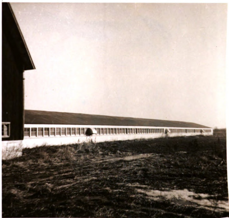
Fig. 47a. Front view of Mr. Joseph Rohmwalter's poultry house, Okemos, Route I, Michigan. Eighty-five windows face south. From left to right: first, second and third fan as referred to in the text. This house is 30' by 200' and contains more than 2000 Leghorn hens.
