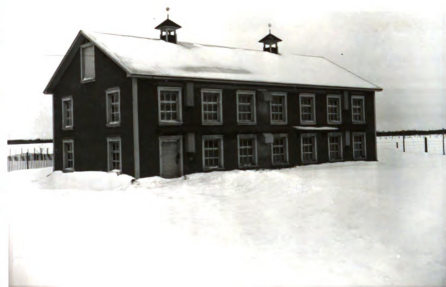
Fig. 62. Mr. Albert Levasseur's poultry house, St. Albert, Province of Quebec, Canada. (Photo furnished by the Shawinigan Water and Power Co., Montreal).
