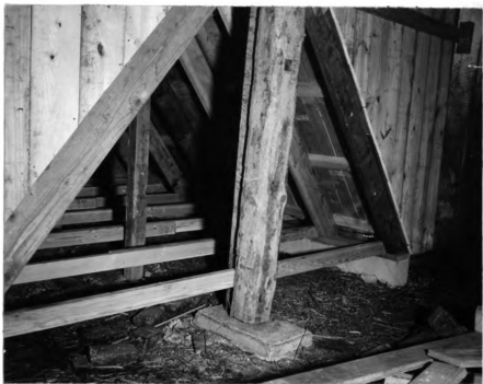
Figure 9. "A" Frame at the Base of Hay Self-feeder for Cattle.
