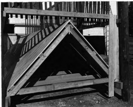
Figure 15. "A" Frame of Hay Self-feeder for Sheep.
