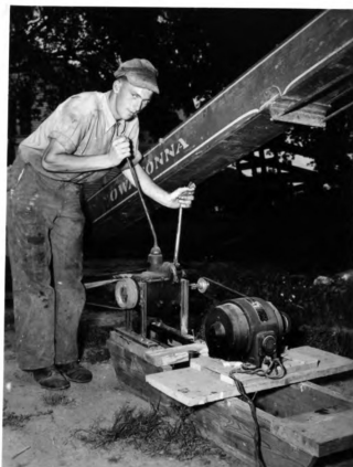
FIG. 62. An Illinois farmer uses a portable motor for the operation of an elevator on his farm. (Courtesy: "Northern Illinois Farm Life" magazine.)
