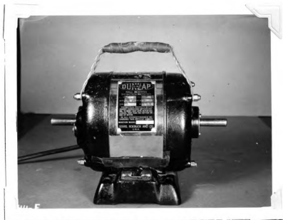
Fig. 22. A portable fractional H.P. motor for a farm home is useful for miscellaneous purposes. (Courtesy: Michigan State College)
