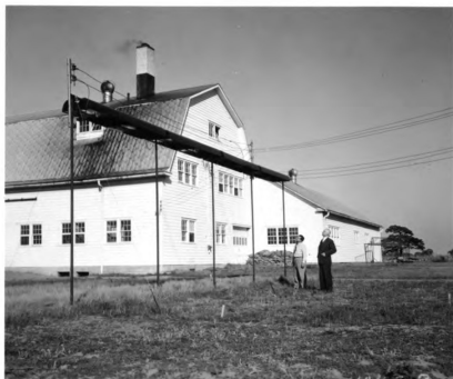
Fig. 71. An experimental electric frost prevention device developed at the Michigan State College. The device consists of two units of heating elements placed under semi-oval aluminum reflectors. The two units are placed alongside each other. Each unit consists of 4 sections placed end to end. The heating element for each unit is continuous (Courtesy: Michigan State College.)
