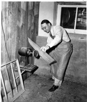
Fig. 49. Cleaning the incubator trays with an electrically driven rotary wire brush. (Courtesy: "Northern Illinois Farm Life" magazine)
