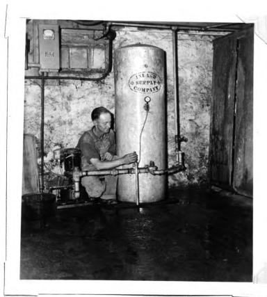
Fig. 8. A water pump provided with automatic switch controls is a great convenience to the farm family. (Courtesy: "Northern Illinois Farm Life" magazine)
