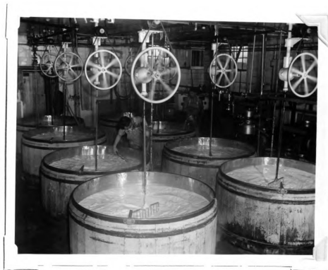
Fig. 34. Electricity is used in cheese making. Notice the small motors operating each of the stirrers. (Courtesy: "Northern Illinois Farm Life" magazine)
