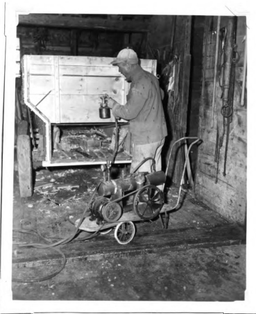
Fig. 66. An electrically operated paint spray used by an Illinois farmer. This unit may be used for pumping (see fig. 63.) (Courtesy: "Northern Illinois Farm Life" magazine.)
