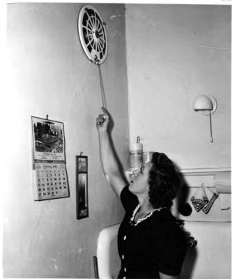
Fig. 13. An exhaust fan removes odors and provides ventilation in the house in warm days. (Courtesy: Northern Life)
