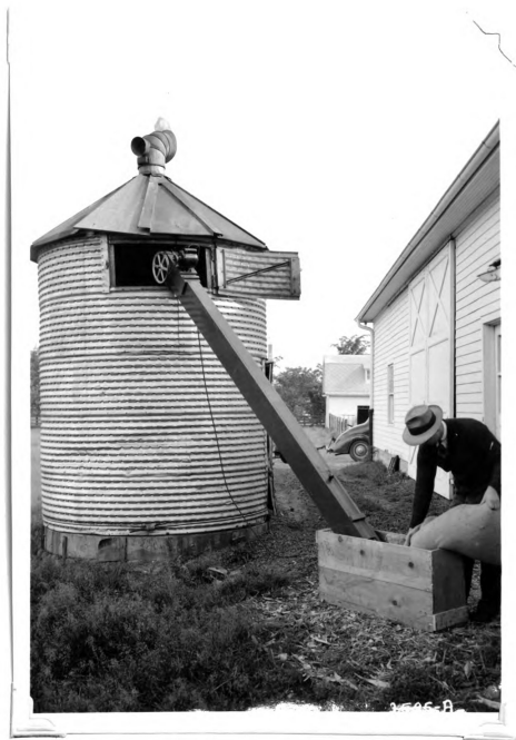
Fig. 40. An elevator operated by a fractional H.P. motor is used in filling the granaries. (Courtesy: Michigan State College)
