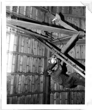
Fig. 44. An Illinois farmer lights his hay mow with electric floodlights. (Courtesy: "Northern Illinois Farm Life" magazine)
