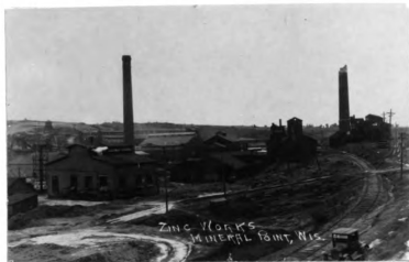
Figure 21. Mineral Point Zinc Company plant. Early 1920's view to the southeast but from a point farther northwest than where Figure 20 was taken. The building in the left foreground with the large stack is the power house. To the left is a part of the plant office. The structure with the partly dismantled stack had been a machine kiln where the jack was calcined. To its left, along the railroad, is the ore receiving and unloading building. (Photo courtesy of Wisconsin State Historical Society. Identification supplied by Mr. Jack Adams, Mineral Point.)
