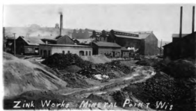
Figure 20. Mineral Point Zinc Company plant. View to the southeast during the early 1920's. The large building in the right-center background with the six steep ridged roof projections held the bag rooms. The roof tops contained side openings to ventilate the building. To the right was the roaster and its stacks. The three small buildings in the center were from left to right: the general warehouse (flat roof), carpenter shop, blacksmith shop. (Photo courtesy of Wisconsin State Historical Society. Identification supplied by Mr. Jack Adams, Mineral Point.)
