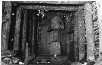
Figure 12. Miners riding in an ore tub. One leg from each of two miner's bodies can be seen protruding from the sides of the metal ore can in the shaft of the Wilkinson mine. Although a dangerous practice, inviting injury, it was commonly engaged in. Note the heavy square set timbering at the shaft base; this was necessary because of the extreme softness of the mine rock. The Wilkinson mine, located just north of Benton, was operated by the Wilkinson and later the Vinegar Hill mining companies between 1909 and 1915. (Photo courtesy of Wisconsin State Historical Society.)
