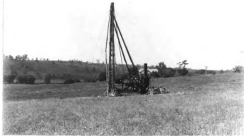
Figure 11. Churn drill. The drill rig, used for exploration purposes, was a common sight in the mining region, especially during the boom periods of the early 1900's. Its utilization helped to place prospecting on a more scientific, as well as a more practical basis. (Photo courtesy of Wisconsin State Historical Society.)
