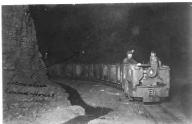
Figure 17. Underground locomotive haulage. Mechanical power replaced man or animal power in the hauling operation in several mines of the period, such as here in the Lawrence mine. This mine, located in the Hazel Green subdistrict, was operated by the Cleveland Mining Company between 1913 and 1917. (Photo courtesy of Wisconsin State Historical Society.)
