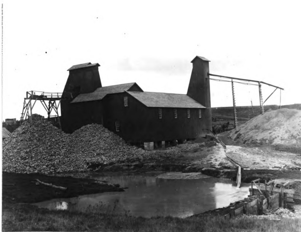
Figure 19. Sunrise mine mill. A typical wooden, level site type of mill structure in the early 1900's. Coarse tailings are at the left, the fine tailings pile is at the right and the mill pond is in the foreground. The Sunrise mine was on a part of the famous Coker ore body, located just north of the village of Rewey. It was opened in 1899 by the Sunrise Mining Company and operated until 1911, after which the property was purchased by the New Jersey Zinc Company, along with several others in the vicinity. (Photo courtesy of Wisconsin State Historical Society.)
