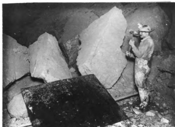
Figure 15. Shoveling from steel plates. The steel plate in the foreground is the type that was usually placed flat on the ground at the end of the haulage track and in front of the working face, to permit easier shoveling. In this picture the worker is about to reduce the size of several large boulders with a sledge hammer before shoveling the ore into cans. The broken material will fall on to the plate on which he is standing.
