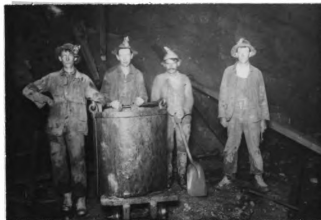
Figure 16. Shovelers at an ore tub. The shovelers or "muckers" were responsible for filling the tubs or cans nearly to the top - they were not filled completely in order to prevent spillage during hoisting and injuring persons below in the shaft. Displayed in the photo are the D handle scoop, pick, and sledge hammer, common tools of the shovelers. Loading was followed by pushing or hauling the cans on low, flat cars to the base of the shaft where hoisting would take place. The job of mucking and tramping was usually paid for on a contract basis - 6 to 10 cents per can loaded and hoisted, enabling good workers to earn $3 to 3.50 per day.
