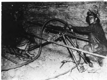
Figure 14. Underground drilling. The common drill used was a compressed air type mounted on a tripod. The limestone rock of southwest Wisconsin did not wear down the bits as fast as the flint in the Joplin district. Still drilling was relatively slow, for the rock is compact and breaks down into a fine powder which is apt to accumulate in the holes when drilling. That difficulty was overcome in part by using water-type hammers which kept the holes washed out as drilling continued.
