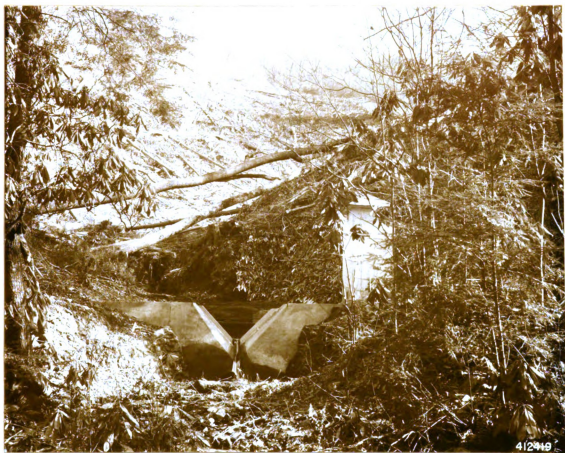
Figure 12. The 90-degree V-notch weir of watershed 17 in February, 1941.
