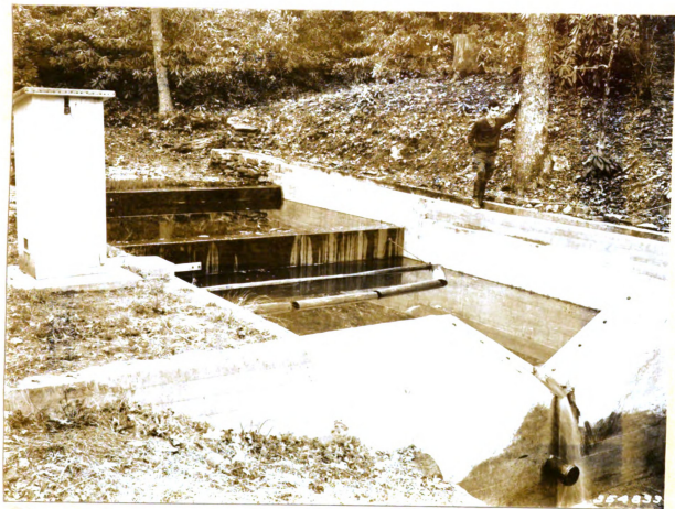
Figure 14. The 120-degree V-notch weir of watershed 18 in September, 1937.
