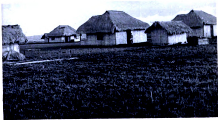
Figure 93. Improved type houses using bamboo for vertical siding at Anak Kamang, Sumba
