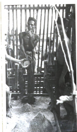
Figure 73. Foot driven grater in small Central Sumatra coconut oil mill with grated coconut meat on floor
