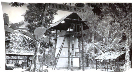
Figure 96. Silo type coral lime kiln near Ambon with capacity of approximately thirty-six cubic feet per thirty-six hour burning period
