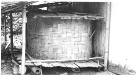
Figure 40. Cylindrical rice lumbung woven from bamboo
