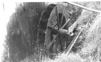
Figure 71. Undershot water wheel for North Sumatra rice pounding mill
