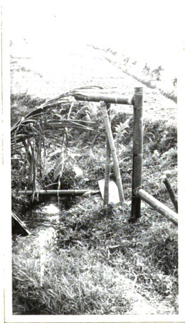
Figure 97. Bamboo pipe showing method of making square joints
