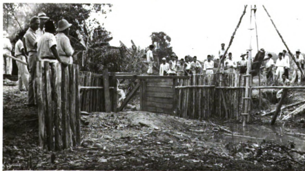
Figure 16. Galam poles used with iron wood in dam construction on Kalimantan
