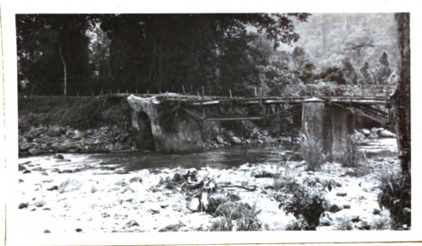
Figure 10. Flood damaged bridge on secondary road in West Central Sumatra
