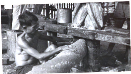
Figure 76. Burlap wrapped meat being fed through wooden geared roller mill
