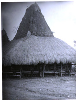
Figure 99. Traditional type of Sumbanese house is with cattle pen in center and platform around pen for living area
