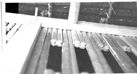
Figure 30. Sago palm frond ribs used as vertical siding in wall construction in Provincial Administrative Office Building in Ambon
