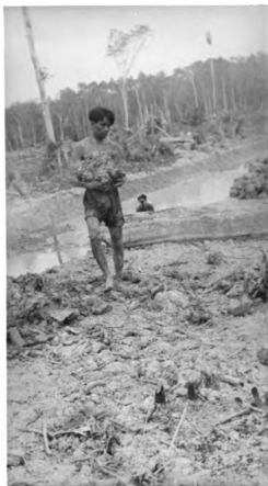
Figure 68. Farmer carrying mud from channel across berm to levee in Mantaran Polder, South Kalimantan
