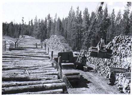
Pictures 43-45 show the railhead at Trude, Idaho, 10 miles west of Yellowstone Park, where Charles Erickson and Son loaded pulpwood for Wisconsin paper mills. Chicken wire around the cars is specified to prevent accidents from logs slipping out enroute.
