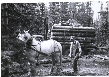
Pictures 41 and 42 show additional loads of lodgepole pine sawlogs loaded by self-loading truck in northern Colorado. The 16-foot and shorter sawlogs were skidded to roadside decks by single horse. The average truckload contained 81 logs and 632 cubic feet. The average time for loading was 89 minutes, and two loads per day were hauled 50 miles to Laramie, Wyoming.
