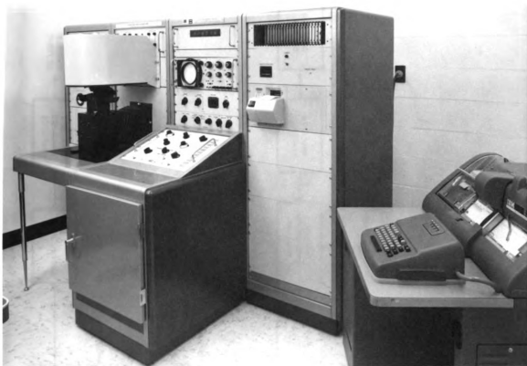
Figure 5. Flying-Spot Particle Analyzer used to determine area cross-sectional areas
