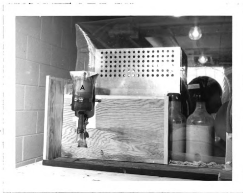
Figure 5. Air-outlet trap attached to rearing isolator
