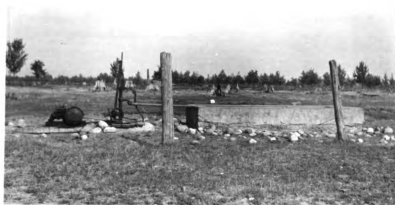
Fig. 15. The gasoline pump and concrete water tank economically furnish good water where lakes, streams or springs are not plentiful.
