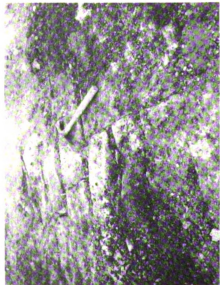
Above: Looking southwest at M 4 5E-M 4 5W, joint set in old quarry. Below: Close up of picture above.
