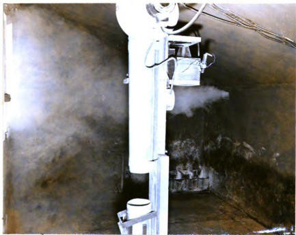
Figure 30. The distribution of the air as it moves across the front of the house towards the air intake of the fan.
