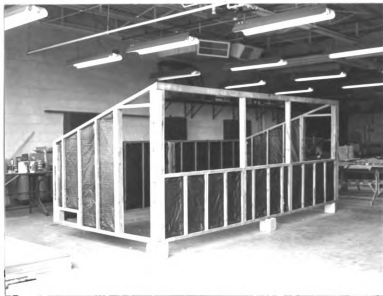
Figure 10. The framework of the houses with the blanket insulation installed.
