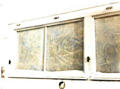
Figure 32. The single-pane windows were covered with frost up to one-eighth inch thick on nights when the temperature outdoors went below 25^{\circ} F.
