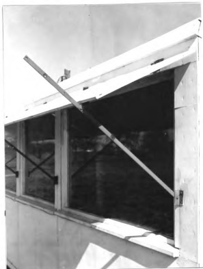
Figure 12. A view showing the windows installed and the sun shades.
