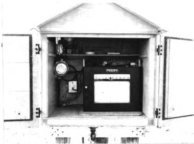
Figure 19. The instrument box for housing the potentiometer, the time clock and the connecting plug.
