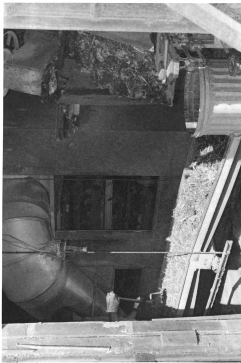
Figure 2.2 Excreta drying tunnel with PVC conveyor belt being loaded with wet excreta.
