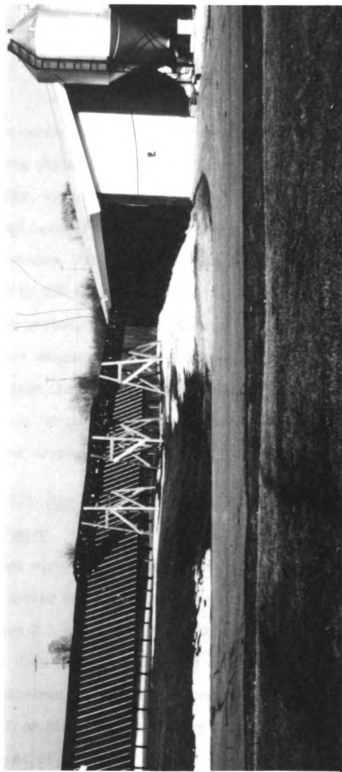
Figure 2.1 View of the solar collector showing air delivery duct for transporting heated air to the poultry house.
