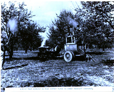
a wind tract sprayer on dual rubber tires is power take-off operated.
