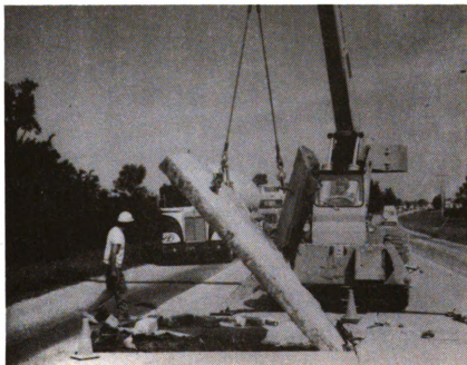
Figure 3-2. Removal of Slab Sections for Joint Repair.
