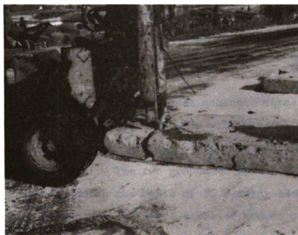
Figure 3-4. Breaking Pavement Slabs for Research Material.
