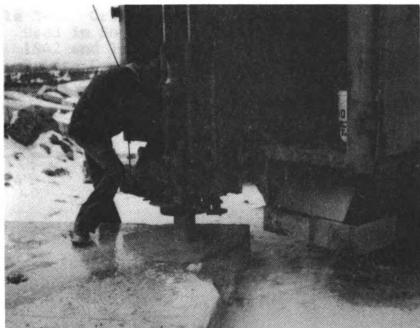
Figure 3-5. Coring Pavement Slabs.
